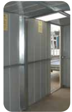
View of portal frame in workshops and garages.
